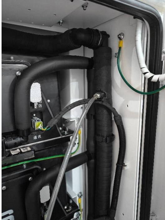
Figure Annex 6- 25 Observe the liquid injection process
