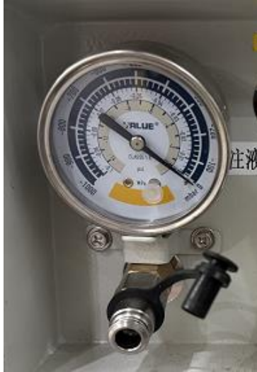
Figure Annex 6- 23 Vacuum pump pressure
