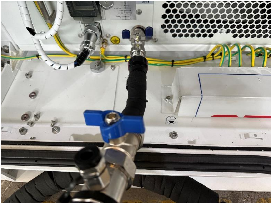
Fig. 9-17 Connect the pipeline of the filling equipment
