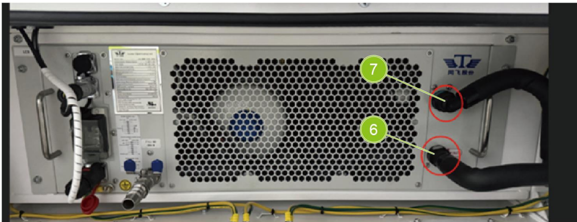
Fig. 9-9 Remove the coolant inlet and outlet pipes
