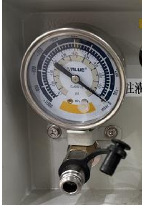
Fig. 9-16 Return water pressure
