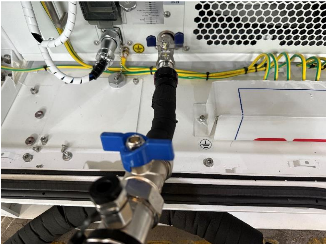
Fig. 9-21 Connect the pipeline of the filling equipment
